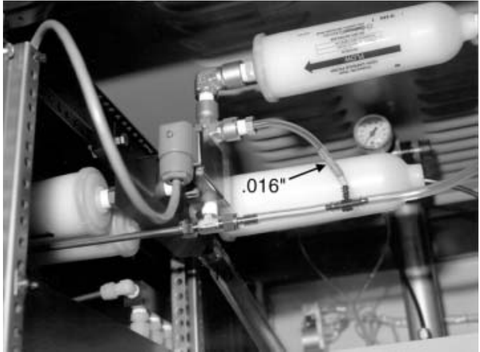
Figure 8-2 Dilution Bridge Showing Orifice
