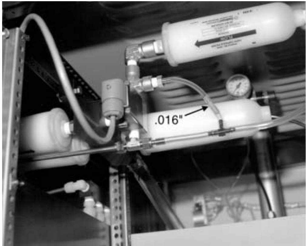
Figure 3-5 The Dilution Bridge
