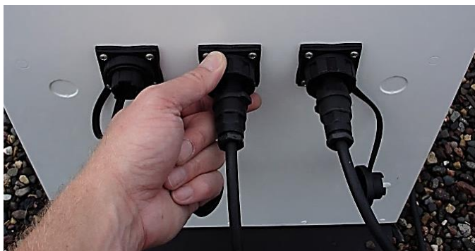
Figure 38: Connect Solar Cells to Battery Enclosure Box
