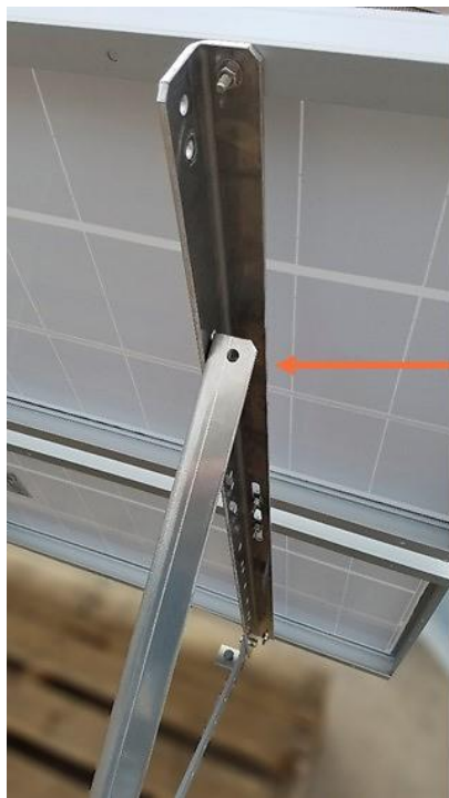
Figure 35: Attach Shorter Structural Angles
