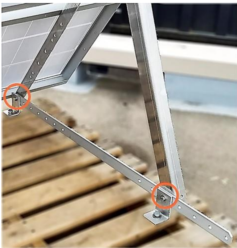
Figure 36: Fasten Two Flat Bar Pieces
