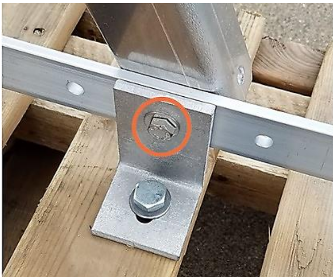
Figure 37: Fasten Mounting Feet
