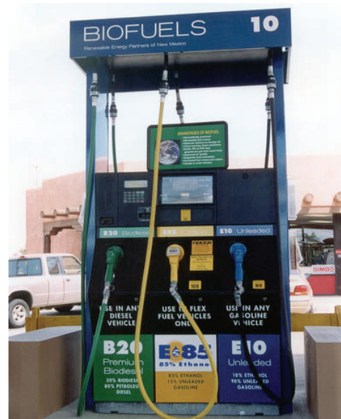
Figure 1: Biodiesel and ethanol fuel dispensing station
