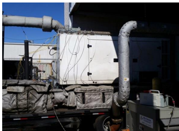
Figure 3: NPET measuring DPF condition of a John Deere 6068TF275 diesel engine stationary generator
