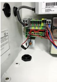
Insert the plastic end of GM460 probe into the sealing gland. Hand tighten the outer nut to create a seal between the gland and the plastic tubing.
