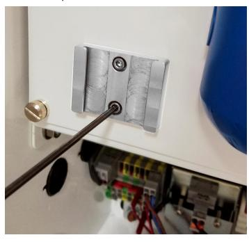
2. Push out the metal plug on the bottom of the enclosure (not shown) and install the sealing gland. The nut should be on the inside of the enclosure.
