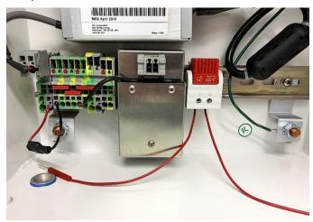
7. Insert the #1 wire from the left side of the Thermostat into the 1st Gray connector.
