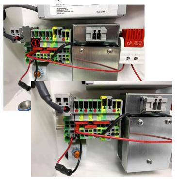
8. Clip the Heater onto the DIN rail.
