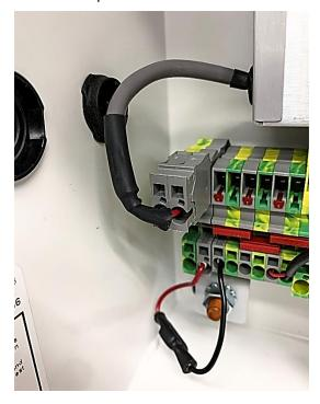
Using a small flat blade screwdriver, install the red wires onto the Thermostat.
