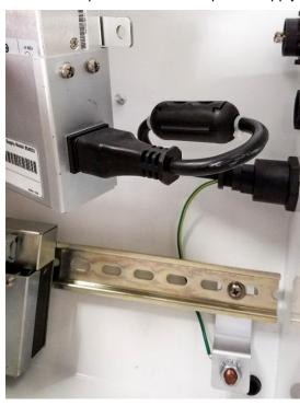
2. Install power supply onto threaded studs.
