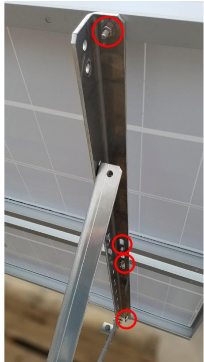
Figure 14: Assemble the Solar Panels on the Mounting Frame
