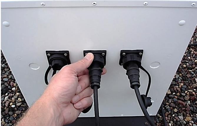
Figure 18: Connect Solar Panels to Battery Enclosure Box
