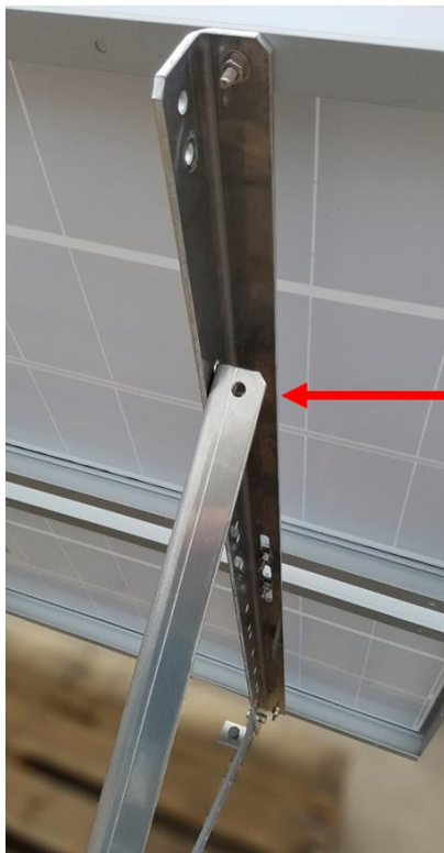
Figure 15: Attach Shorter Structural Angles
