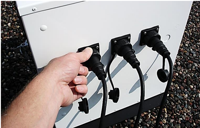
Figure 20: Connect Power Cable to the Environmental Enclosure
