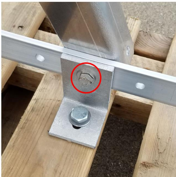
Figure 17: Fasten Mounting Feet
